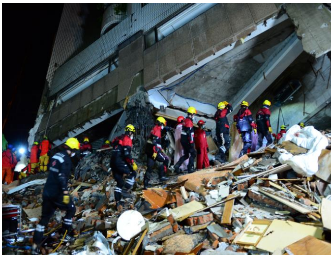
救災隊進入雲門翠堤大樓搜救
